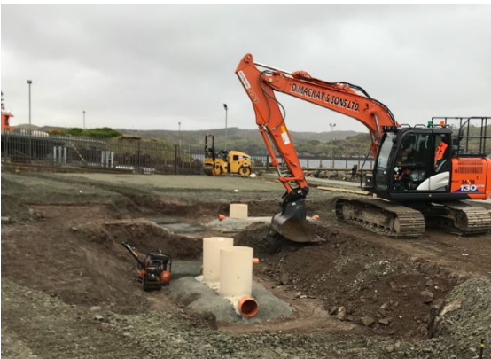
Drainage installation in progress
