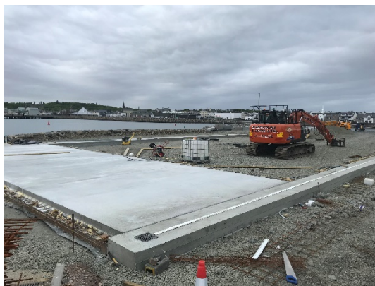
Concrete slab part-complete
