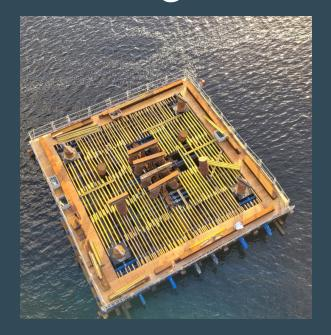
The temporary support (formwork) for the concrete deck is being installed. Once complete, the concrete to form the deck will be poured in four layers. Each layer will be 1m thick.
