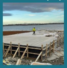
The contractor has started to install the reinforced concrete slab at the junction of the two quays.
