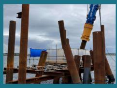
Installation of the 16 berthing dolphin piles was completed in August.
