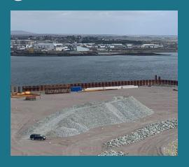
Sub-contractor Breedon is crushing rock blasted from the site for use as a gravel surface material on the reclamation area.
