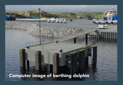
Work will start in May on construction of the berthing dolphin. This is located 60m to the south of the main quay. It measures 15m x 16m on plan and will allow vessels over 300m long to berth at the main quay.
