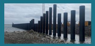
The contractor has installed the final tubular piles at the linkspan quay. As these are founded on rock, the piles must have rock anchors installed. This process involves a hole being drilled into the rock seabed at the bottom of the steel pile. Following this, the rock anchor is installed and grouted into the seabed and the bottom of the pile.
