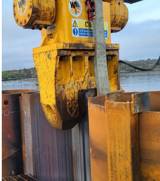
King pile being driven into the seabed, left, and sheet pile being driven into the seabed, right
