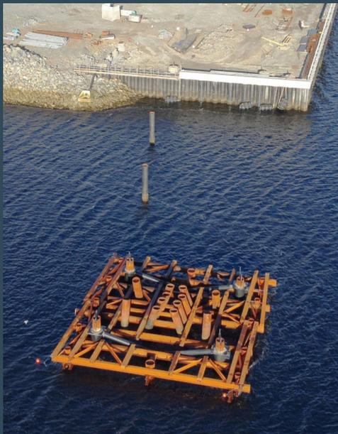
A berthing dolphin is being constructed to the south of the main quay, to allow long vessels to berth.
