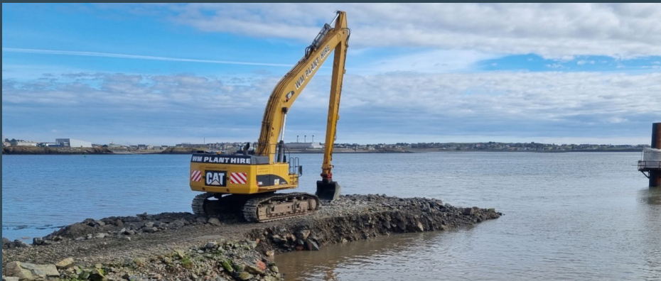
Working platform for completion of linkspan quay wall under construction
